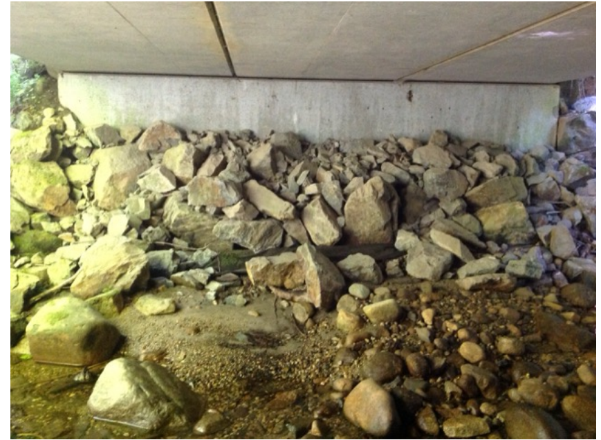
Right Bank Abutment when facing downstream
