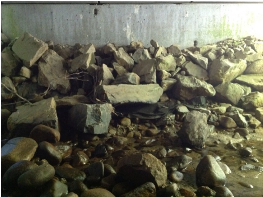
Left Bank Abutment when facing downstream
