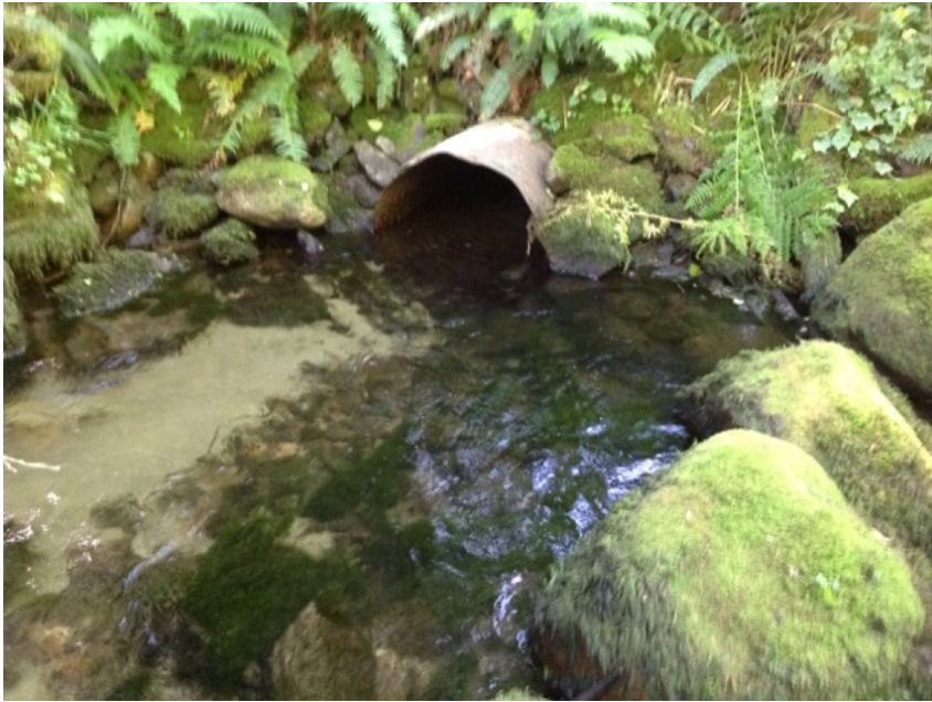
channel being diverted through 900mm CSP, taking 80% of the flow
